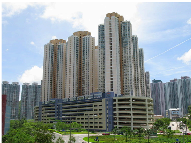
Figure 1 (Left): A typical podium-type development with 11 residential towers sitting on a 7-storey carpark. (Source: Wikipedia user / Baycrest. License: CC-BY-SA-2.5). Figure 2 (Right): Diagram explaining the permeability of buildings requirements. (Source: Hong Kong Buildings Department.)
